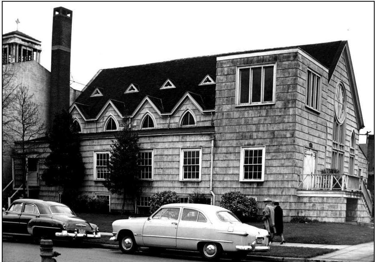
Rose City Park's Original Building as seen during the 1950s.
